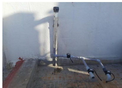
Figure 3 Water Pipeline Connection System
